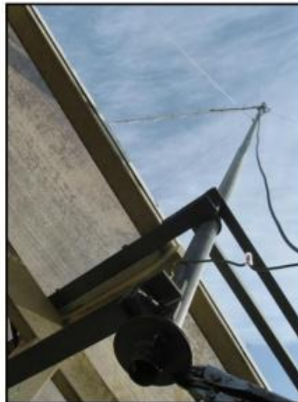
ALL HOME BREW MAST AND ROTATING SYSTEM WITH LOWERING SLIDE ARRANGEMENT
