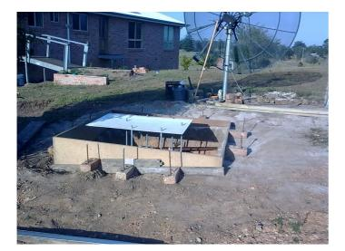
A cement sheet provided the template for the stud alignment and kept them in the right place during the pour and setting of the concrete.
