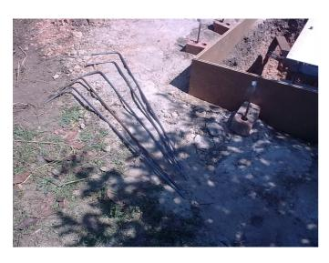
Extra steel starter bars were also ready to be placed into the wet concrete to further tie in and reinforce the whole tower base.
