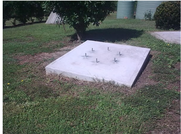
The cured base now without the stud template.
