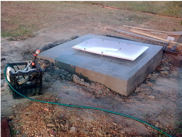
Concrete base poured and levelled.
